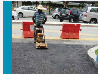
▲ STEP 03 Compact * With hand tamping / machinery or self compact by passing vehicle
