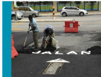
▲ STEP 02 Lay & level material
