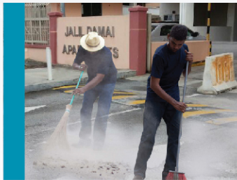
▲ STEP 01 Clean & clear targeted repairing area
