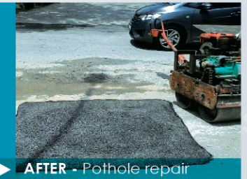
▲ STEP 04 Open for traffic immediately * Open for traffic even it rains right after complete of installation
